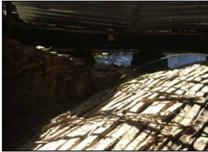
Figure 2: Part of the roof of the meqdes Source: Photo Marshet Girmay, 2016.
